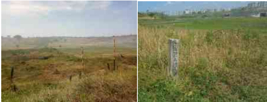
Figure 4: TAZAMA pipeline infrastructures close to the project site
